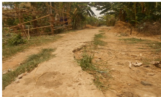
View of CC road in Beluria GP under Pattamundai PS damaged without cut off
