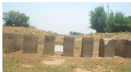
View of check dam in Jari GP under Binjharpur PS where catchment area is higher than the CD height
